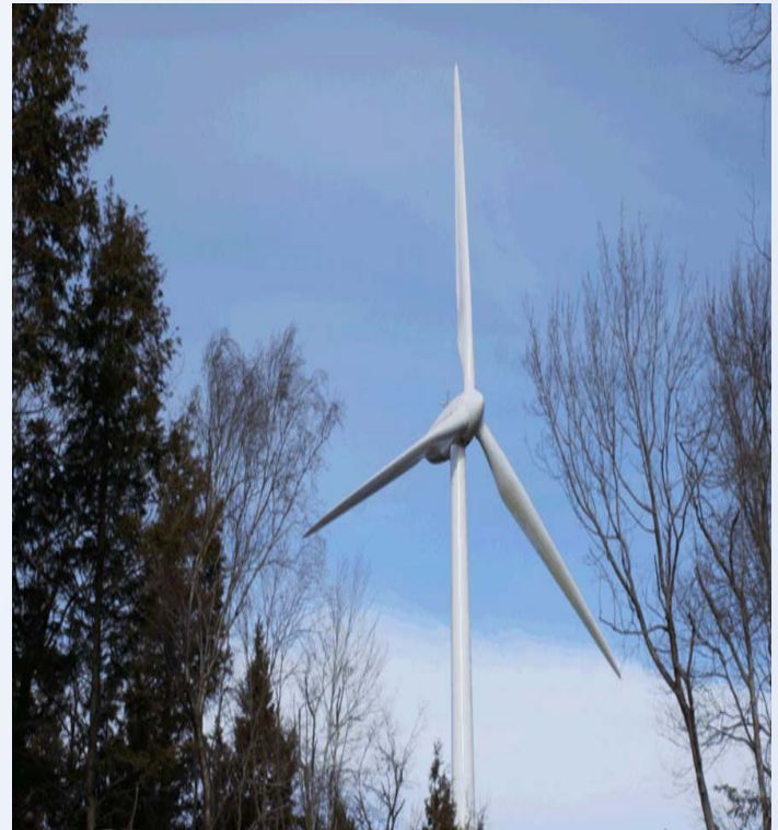
Berkshire East Ski Area's 900KW Wind Turbine
