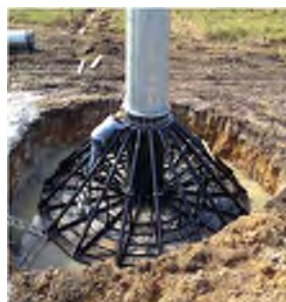
Figure 3-5. Prefabricated foundation installed by Skylands Renewable Energy
