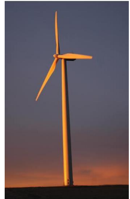
Rosebud Sioux's (SD) Little Soldier Turbine (First 750-kW turbine on tribal lands in contiguous United States)
