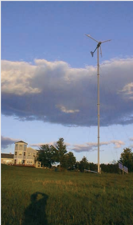
FIGURE 3 Bergey Excel 10, an 8.9-kW turbine at a residence in Vermont
