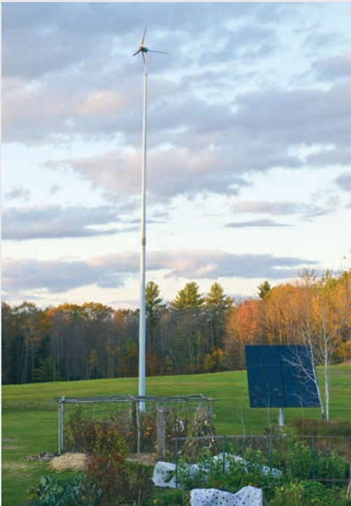
FIGURE 2 Distributed wind turbine at a residential site in Maine 1.8-kW Pika Energy turbine
