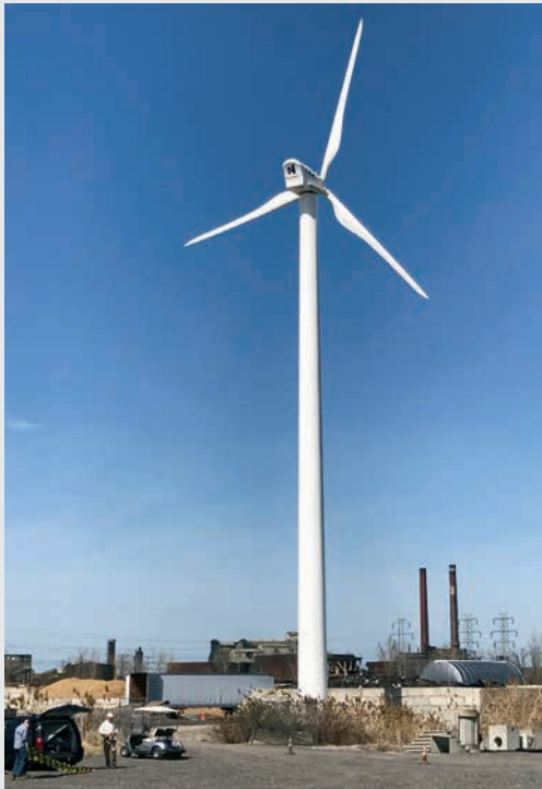
FIGURE 4 A 100-kW Northern Power Systems turbine at the Triad Recycling Facility in New York
