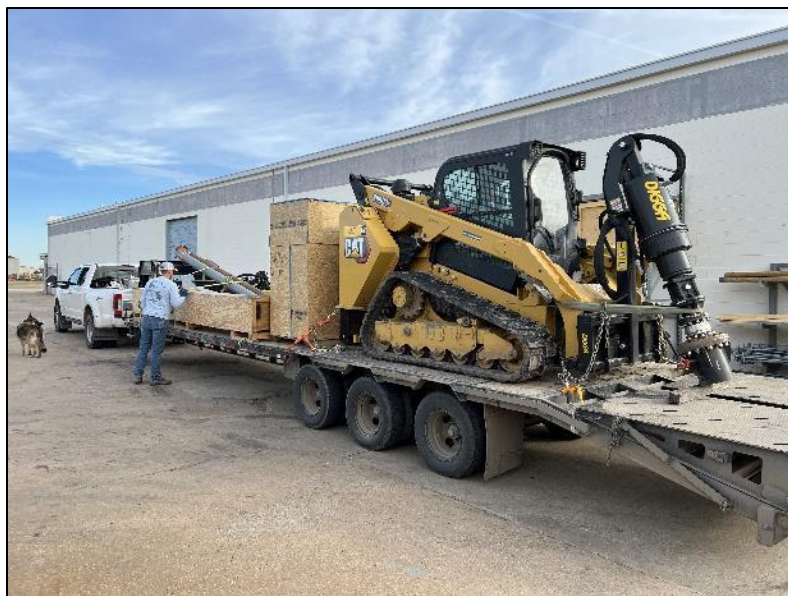
Skid-Steer with Helical Anchor Rig
