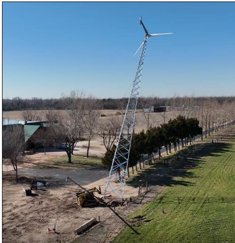
Tilt-up Tower on Helical Anchors
